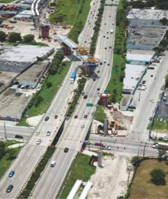
Balanced cantilever construction over SR 112 that required a main span of 256 ft. Photo: URS Corporation.
